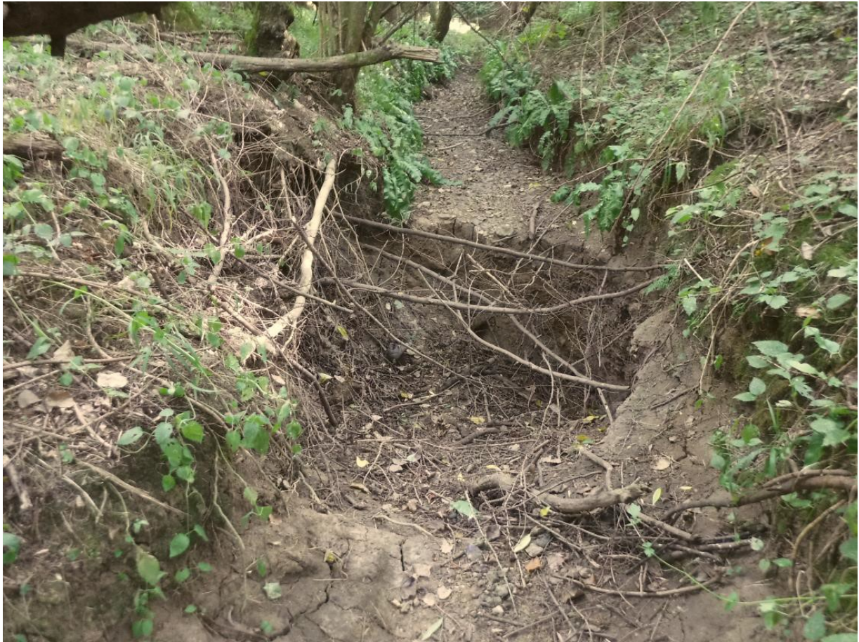
Figure 17. Looking downstream at Claypit Gully Sink. Collapse feature just downstream of dry weather sink. Photo by A. Farrant.
