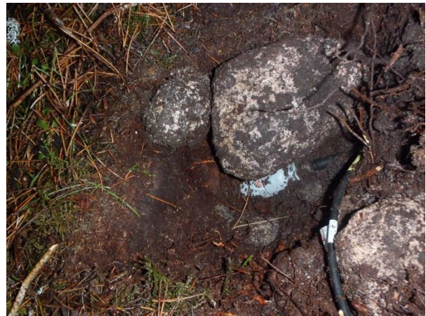
Soil moisture sensor installed below a tree in the plantation forest area
