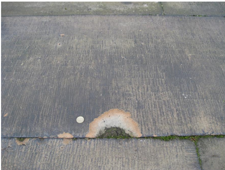
Fig. 16. Detail of paving slab showing tooled surface, detailed as a series of droved bands. The damaged edge reveals the stone to be a pale grey/cream coloured sandstone weathering to a strong orange surface patina, typical of local Edinburgh sandstone such as Hailes. Donaldson's Hospital (3204)
