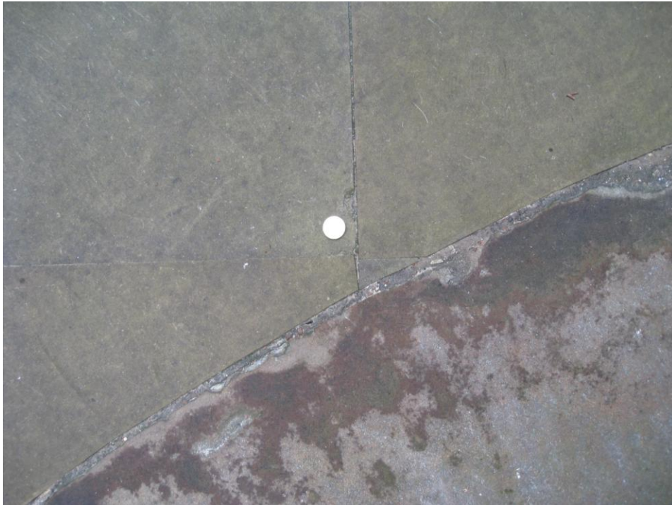
Fig. 33. Detail of junction between original curved steps (Hailes-type sandstone) and replacement 'York-type' sandstone flags. The York stone has a more uniform greyish colour compared to the orange-red patina on the Hailes sandstone. New College (3111)
