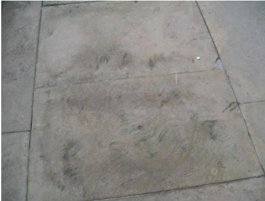
Fig. 3. Typical 'contour' surface pattern of paving slab in Old College, caused by the presence of ripple-bedding in the sandstone. This distinctive texture, and the associated variable colour, is typical of Hailes sandstone (see section 9 for full explanation). (3070)
