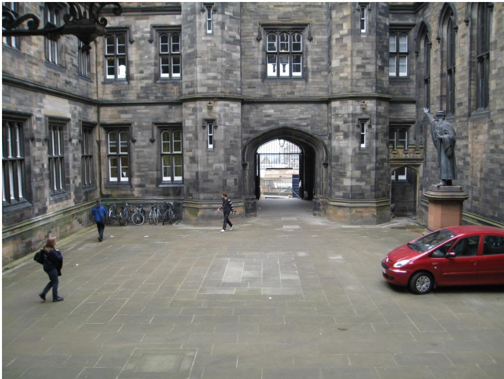
Fig. 30. General view of courtyard showing rectangular centred paving pattern. New College (0912)
