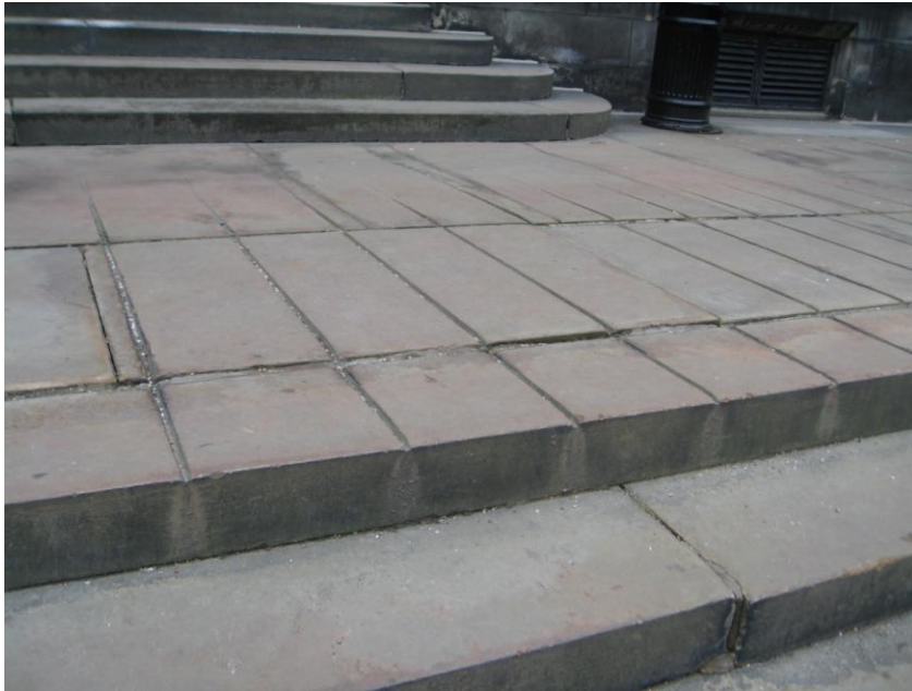
Fig. 11. Terrace pavement adjacent to steps leading down to gravel courtyard (south side of quad), showing narrow channels cut into pavement to provide drainage allowing rainwater to flow down the steps. This tooling (present in a number of places on the terrace), is presumably not part of the original paving design and was undertaken retrospectively to improve drainage. It is disruptive to the uniform paving pattern. (0898)
