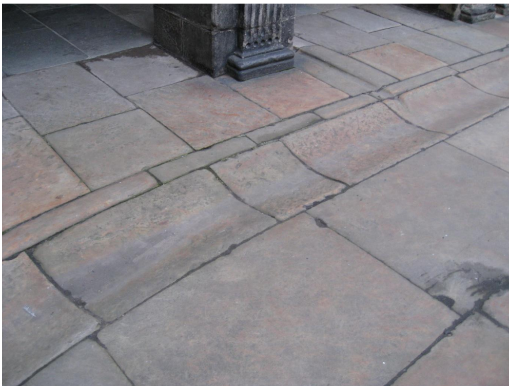
Fig. 24. Details at edge of central courtyard showing dished gutter with outer kerb, all made from Hailes-type sandstone. The kerb blocks are bedded on edge. George Heriot's School (3250)
