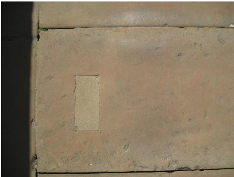
Fig. 2. Detail of original paving slab of Hailes-type sandstone showing indent repair using northern England ('York-type') sandstone, highlighting the contrasting coarse grained 'gritty' texture and bland buff colour compared to the original Hailes stone (3450).
