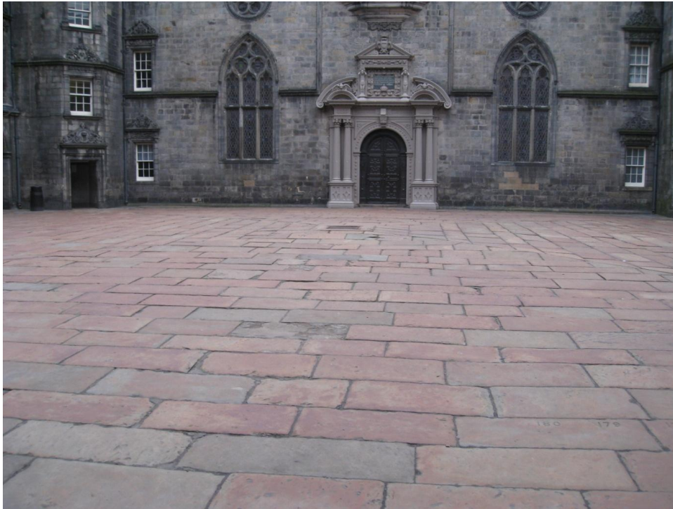
Fig. 19. General view of central courtyard showing rectangular centred paving pattern with strong variable orange-brown patina to flagstone slabs, typical of Hailes-type sandstone. The pavement shows a gradual fall in height from centre to margins to allow drainage of water. George Heriot's School (3234)
