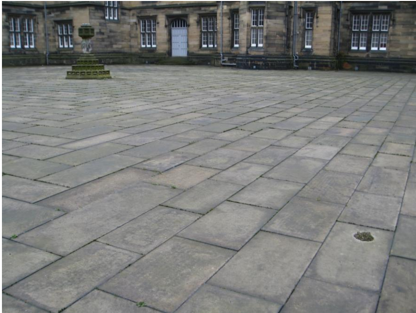
Fig. 15. General view of flagstone paving in central courtyard, showing centred rectangular paving pattern with central fountain. The flagstone is sandstone with a variable orange-brown surface patina (rather dull due to biogenic soiling). The pavement shows a gradual fall in height from centre to margins to allow drainage of water. Donaldson's Hospital (987)
