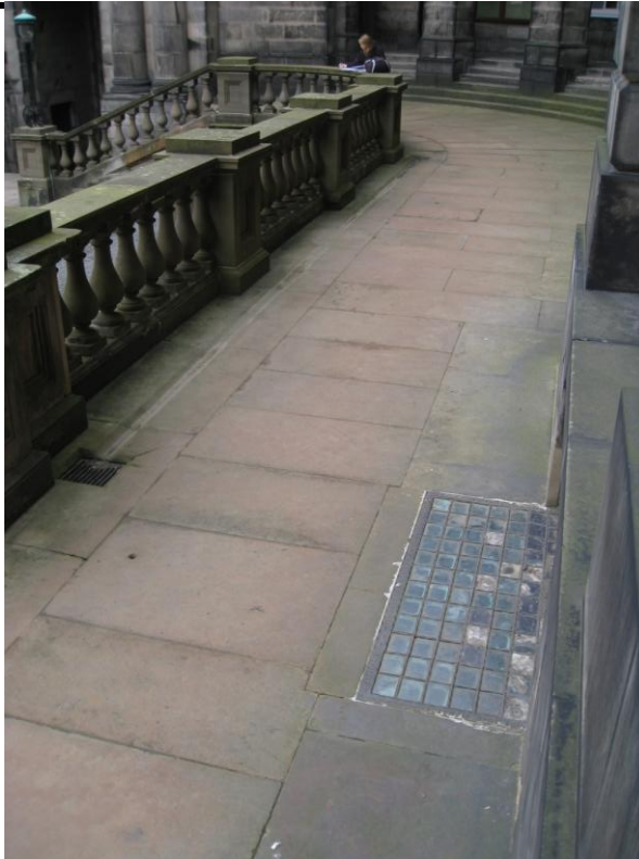
Fig. 5. Southeast corner of the terrace pavement, illustrating the three main paving components described in the text (Narrow area in the foreground; Wide area in centre of image; Curved corner at back). (3080)
