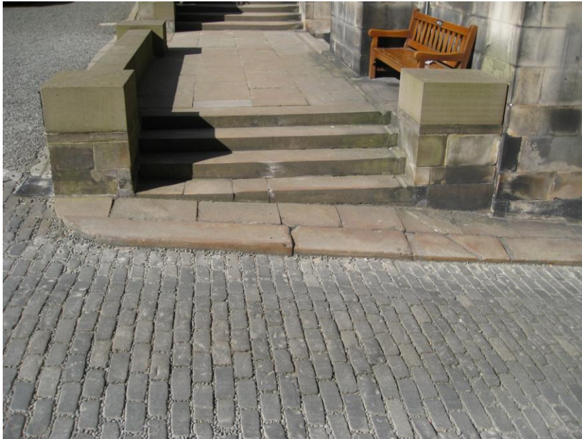
Fig. 13. Inner part of vehicle entrance to Old College, showing dark whinstone setts against original Hailes-type sandstone pavement (note distinctive orange-brown patina). A drainage channel has been cut diagonally across the pavement below the right-hand side of step. Note also the large 'recent' replacement copestones on the terrace wall using a grey-buff Northern England sandstone, giving a 'blocky' appearance uncharacteristic of the Playfair detailing. (3431).
