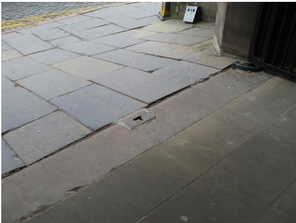
Fig. 34. Entrance to New College, showing a mixture of three types of paving stone. The long entrance sill is the original Hailes (or Craigleith) type stone; the courtyard (bottom-right) has been repaved using a greenish-buff York-type sandstone; and the external pavement has been paved using 'modern' dark grey Caithness flagstone.
