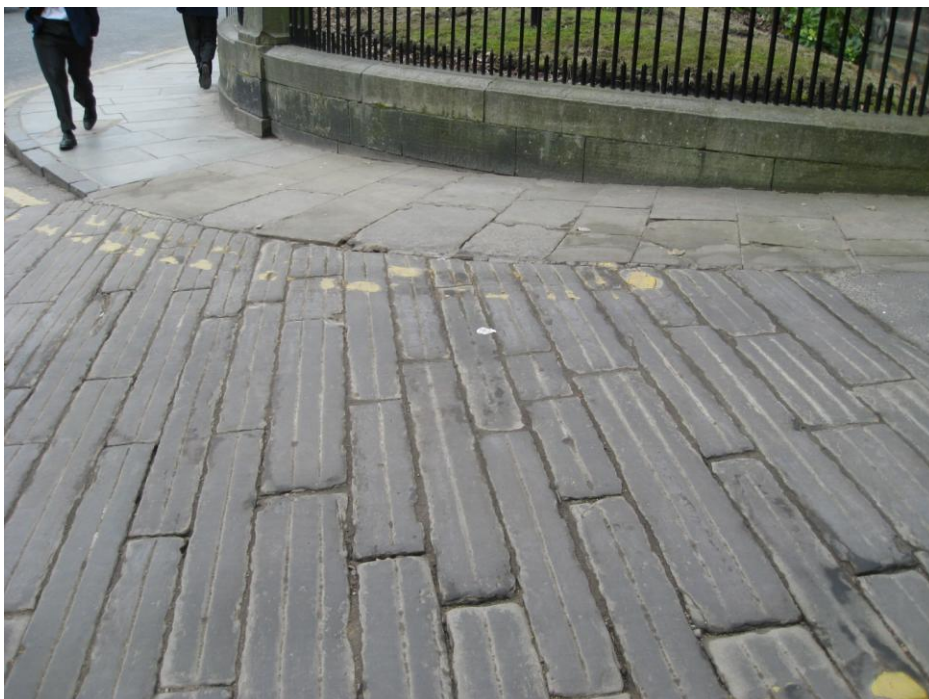
Fig. 28. Entrance to George Heriot's School on Lauriston Place consisting of elongate sandstone blocks on edge, each with a simple coarse groove cut along the length of the block, probably to prevent skid. The stone appears to be a Hailes-type sandstone, the same as that used in the courtyard. George Heriot's School (3087)
