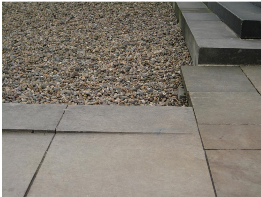
Fig. 43. Part of recently paved area (Clashach Sandstone) showing well-executed edge detailing for sloping footpath. National Galleries (3139)
