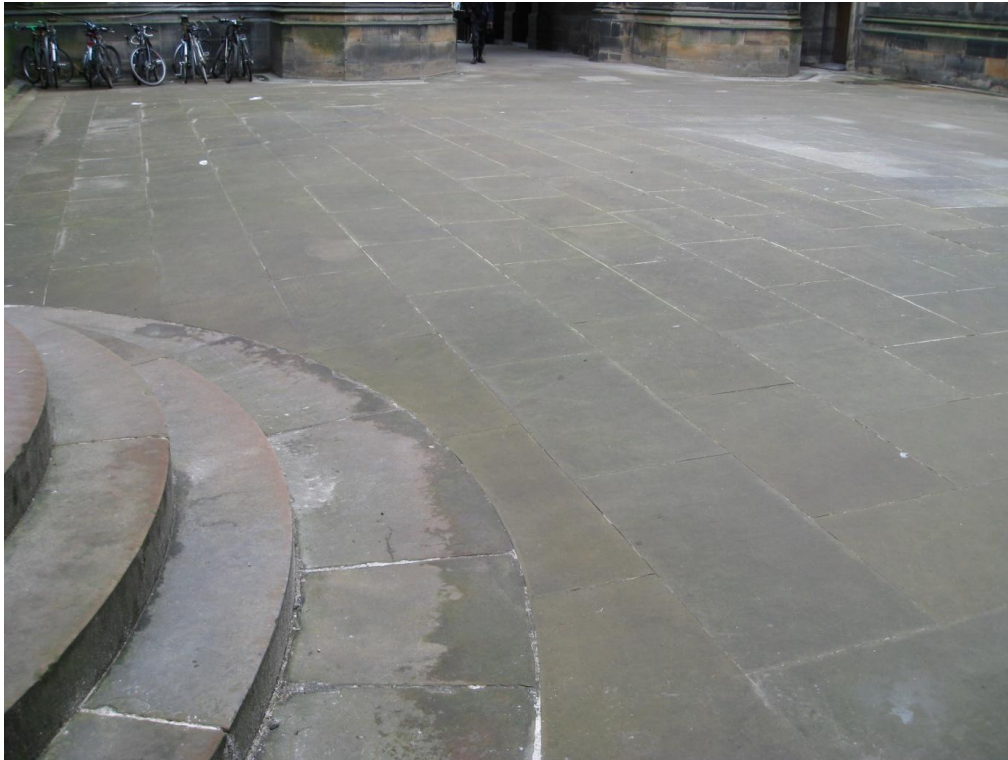
Fig. 29. Edge of curved entrance steps showing junction with replacement courtyard paving. New College (3104)
