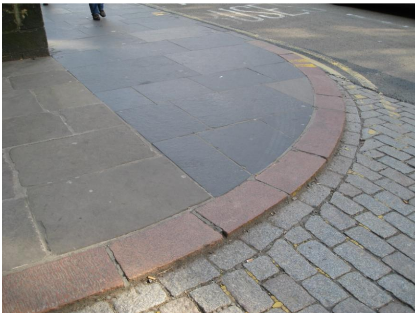
Fig. 14. Entrance to Old College at South Bridge, showing 'modern' dark blue-grey Caithness flagstone on the public pavement adjacent to the paler original Hailes-type sandstone paving of Old College. The vehicle entranceway comprises grey granite setts with wide kerbstones of pink Corrennie (Aberdeenshire) granite. (3444).
