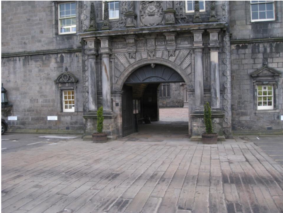
Fig. 27. North entrance to central courtyard showing stone paving on roadway, consisting of elongate sandstone blocks on edge, each with a single centre groove cut along the length of the block. The stone appears to be a Hailes-type sandstone, the same as that used in the courtyard. George Heriot's School (3230)
