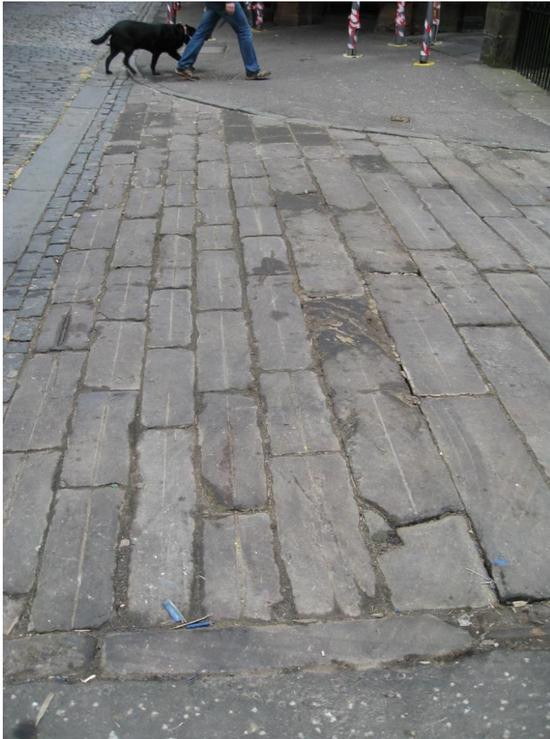
Fig. 37. Part of vehicle entrance to New Register House with sandstone blocks laid on edge, each with a simple tooled groove cut along the block length. This pattern is almost identical to George Heriot's School (Figs. 27 and 28) (3184)
