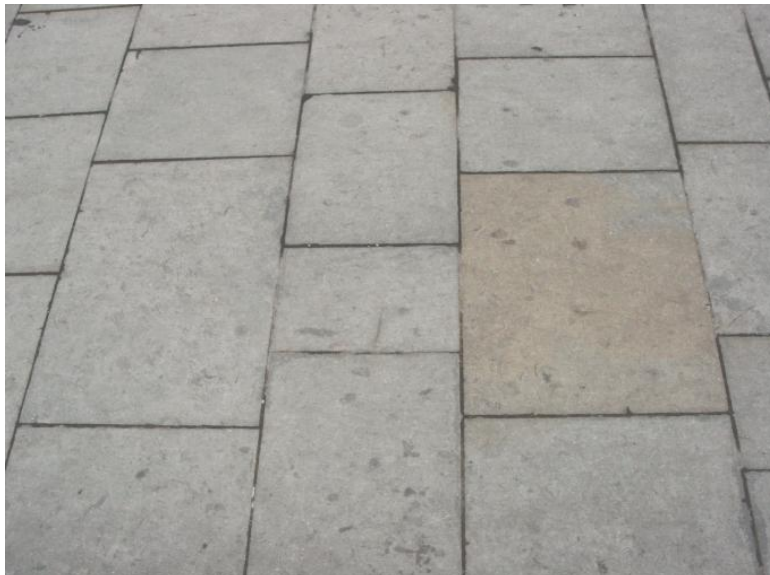
Fig. 51. Modern natural stone pavement on Waverly Bridge, typical of sandstone from Scout Moor quarry. This stone type has some similar characteristics to historic Hailes-type sandstone paving used in Edinburgh, in particular a variable colour from pale grey to orange-brown and the presence of bedding planes on the surface providing a 'contour surface' effect.
