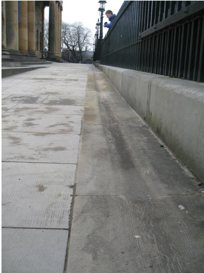
Fig. 42. Replacement sandstone paving showing dished gutter at edge, with hand-tooled droved surface finish. National Galleries (930)
