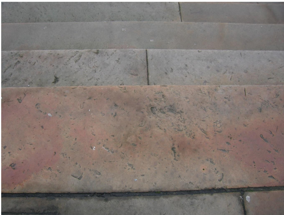
Fig. 34. Detail of entrance steps to General Register House showing characteristic variable orange-red patina and 'contoured' natural surface texture, all typical of Hailes sandstone.
