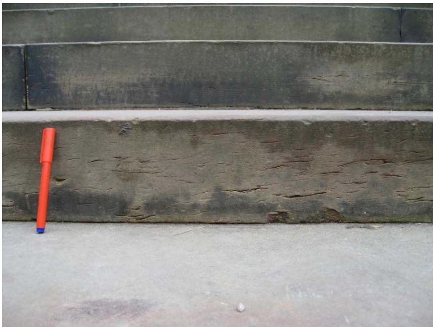
Fig. 4. Detail of step showing the presence of ripple bedding (small irregular discontinuous bedding planes) in the sandstone. This is typical of Hailes sandstone (and also some Craigleith sandstones), resulting in the distinctive 'contour' pattern to the slab surface. The same 'Hailes-type' sandstone appears to have been used for both the steps and paving at Old College. (3056).
