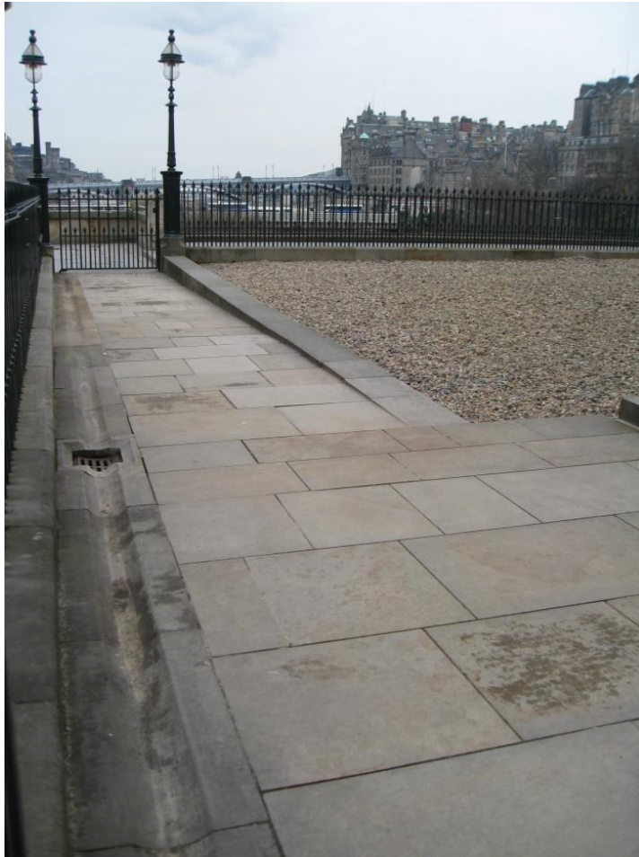
Fig. 40. General view of recently paved area showing new flagstone footpath, edging to gravel area and dished gutter, all using Clashach sandstone. Note the variable colours in the flagstone paving which resembles historic Hailes sandstone paving. National Galleries (935)
