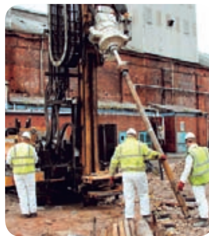
Installation of a borehole monitoring network at a contaminated site.
