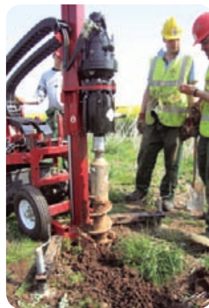
Drilling rig operation training.
