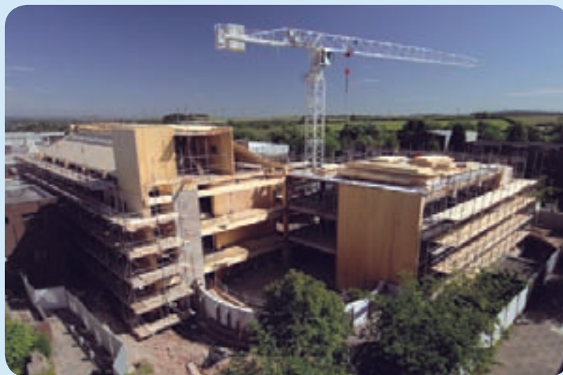
Construction of the William Smith Building, Spring 2008.
