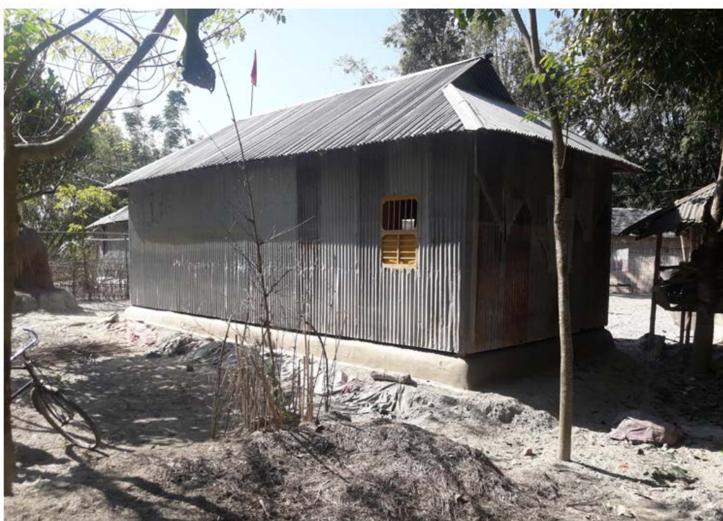
Figure 1 Reconstructed home on a raised plinth after flooding in Bangladesh © 2017 Beth Simons
