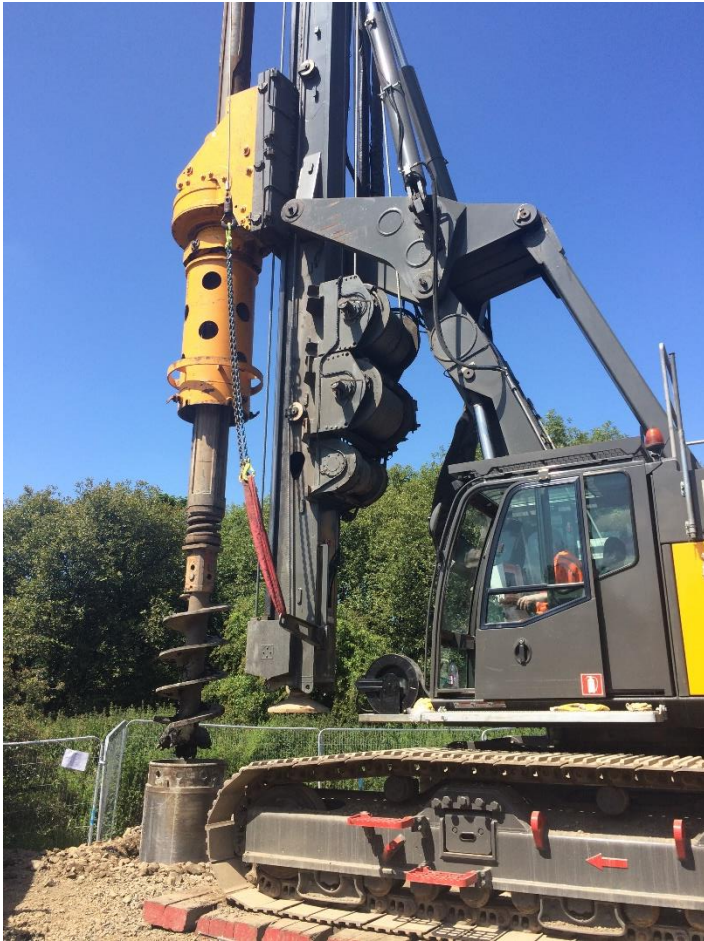
Figure 5 The piling auger rig drilling the made ground-superficial section at GGA09r
