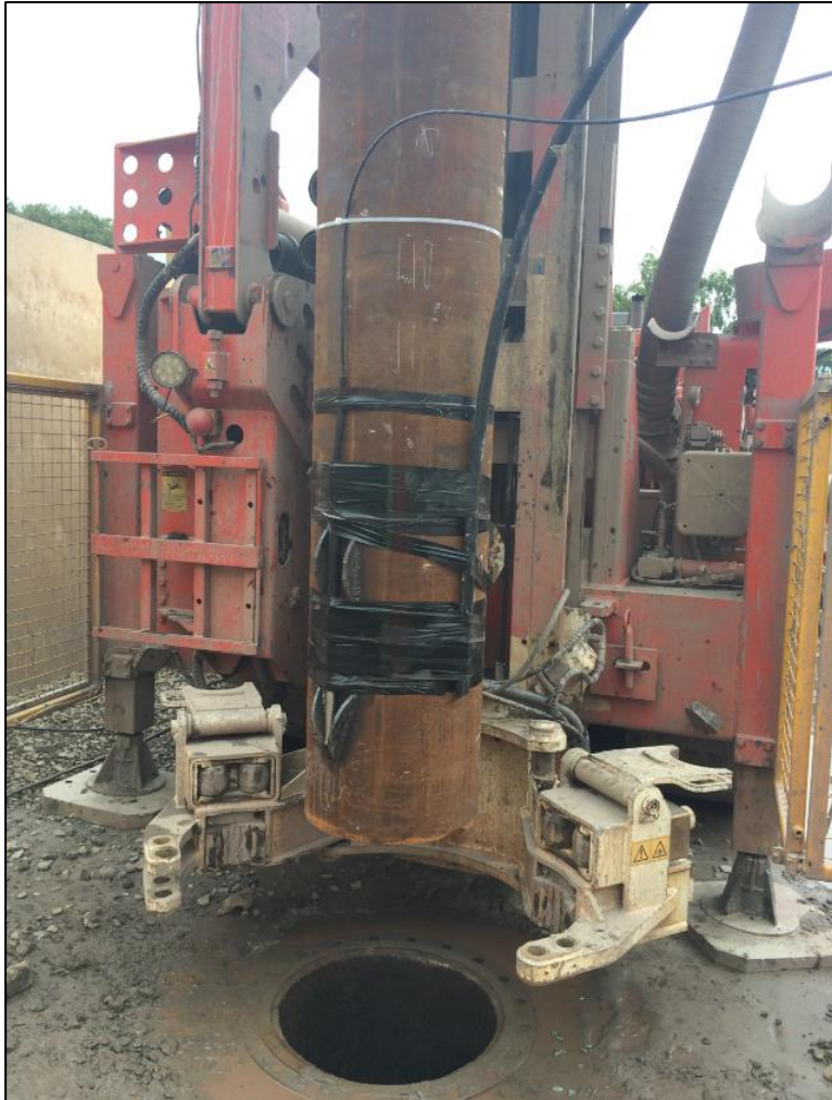
Figure 5 Photograph of the bottom section of the steel superficial deposits casing with fibre-optic cable attached and welded centraliser, during installation at GGA02 on 18/07/2019
