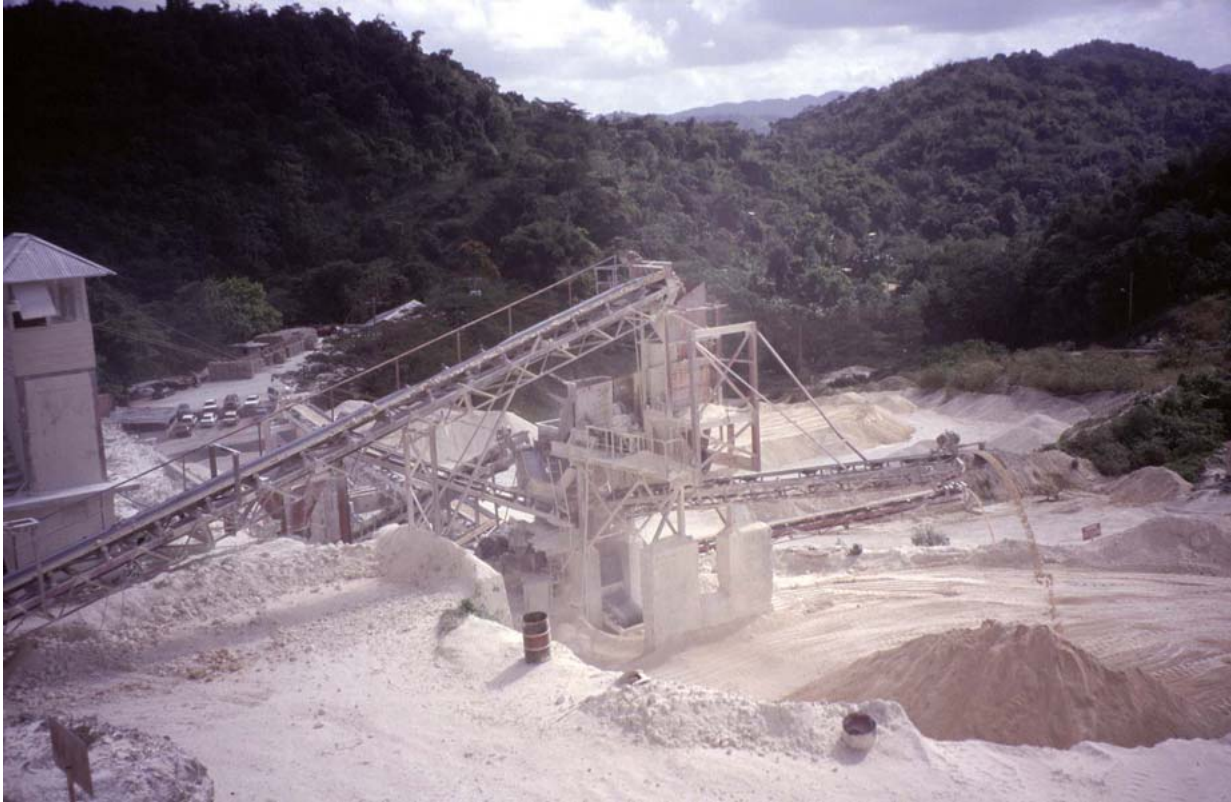
Figure 11 Limestone processing plant, John's Hall Aggregates, near Montego Bay, Jamaica.
