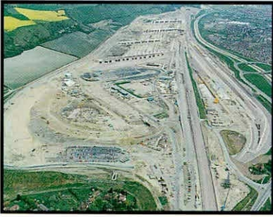
Figure 39. Folkestone Terminal site under construction. (Copyright Eurotunnel courtesy of QA photos).
