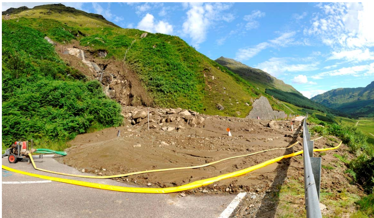
Figure 6 Landslide deposit blocks the road on the A83 Rest and Be Thankful Pass in August 2012
