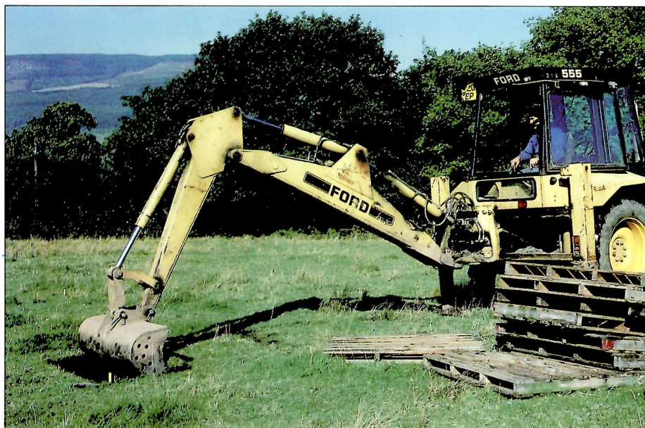
Plate 43. Turf being stripped from the donor site before being transported on pallets to the receiver site – October 1990
