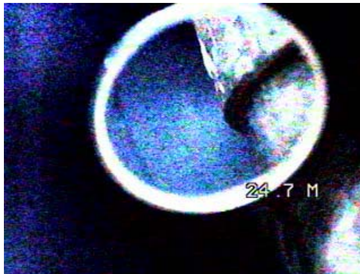
Figure 7. Steel rising main in the Gasory borehole
