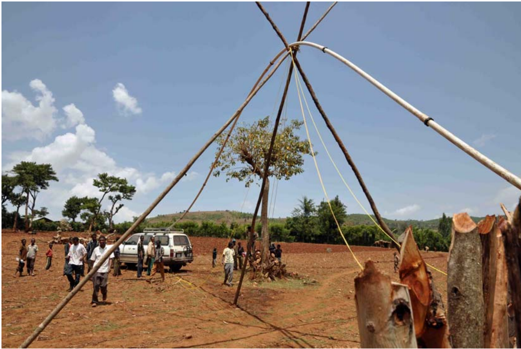
Figure 10. Removing the PVC riser
