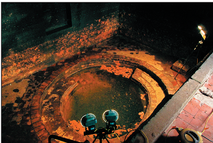
Figure 3: The brick-lined well within the Taffs Well spring's well-house.
