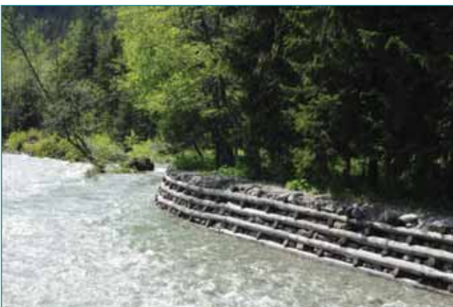
Tree trunk and boulder bank revetment.
