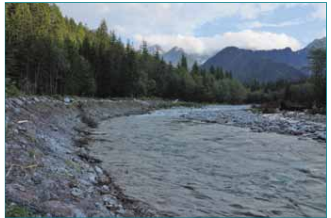
Re-profiled bank with wire basket gabions.
