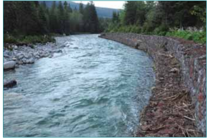
Bank reinforcement on the Biela voda downstream of our survey sites.
