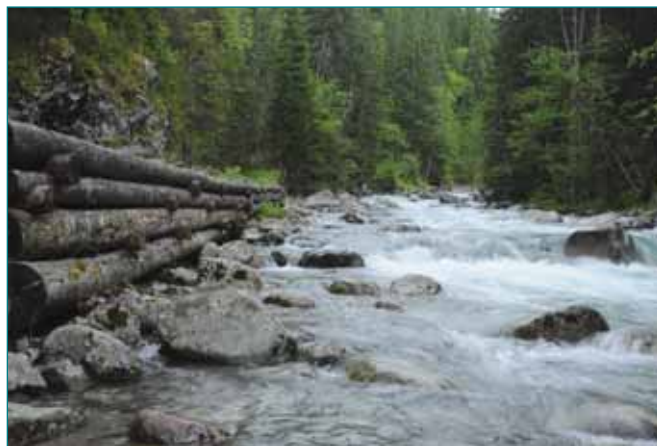
Artificial bank reinforcement and reprofiling produces a high HMS score.
