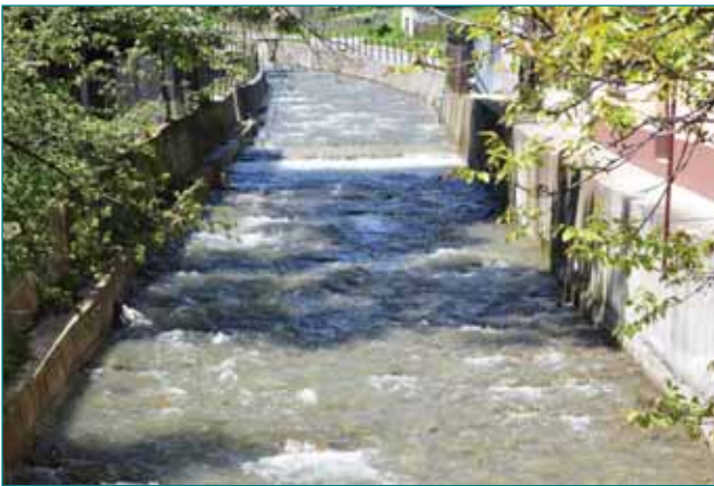
Concrete banks-an extreme form of channel modification.
