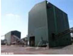
Photo 27. Plant containment buildings
