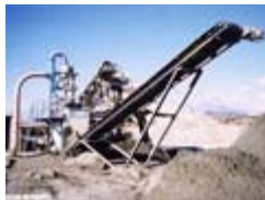
Photo 24. Mobile washing plant
