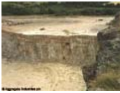
Photo 27. Before hard rock blast
