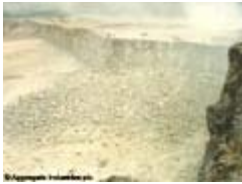
Photo 29. After hard rock blast
