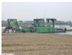
Photo 39. Sand and gravel dredging
