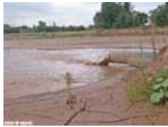
Photo 26. Discharge into silt lagoon
