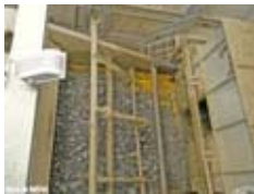
Photo 59. Dry screening crushed rock
