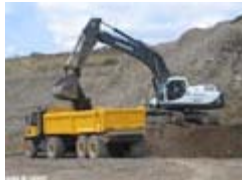
Photo 34. Loading with backhoe
