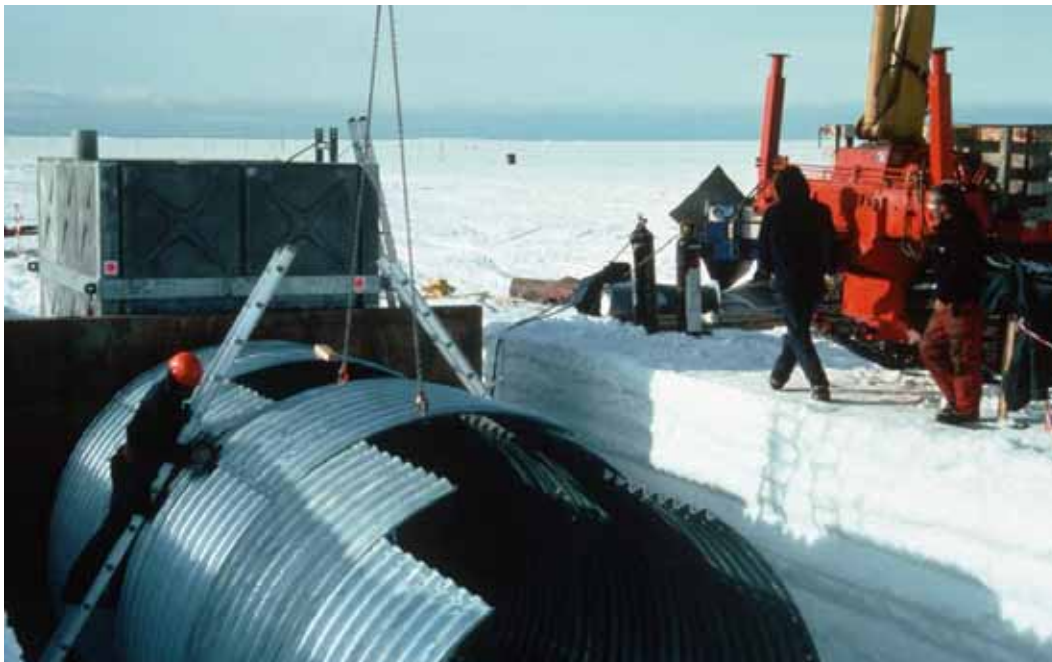
Figure 15. Laying the ARMCO steel tunnels on the snow surface in 1991/92
