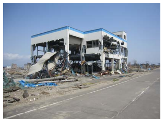
Figure 3 Photograph of tsunami destruction – Yagi Port (Photograph by D. R. Tappin 2011).
