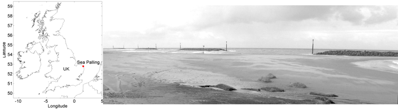
Figure 1. Location map and view of the Sea Palling breakwaters looking north from the slipway. The first phase of four breakwaters are clearly visible together with the tombolo linking to the nearest at low water. The radar was located a few metres from this position up on the flat roof of a lifeboat station.
