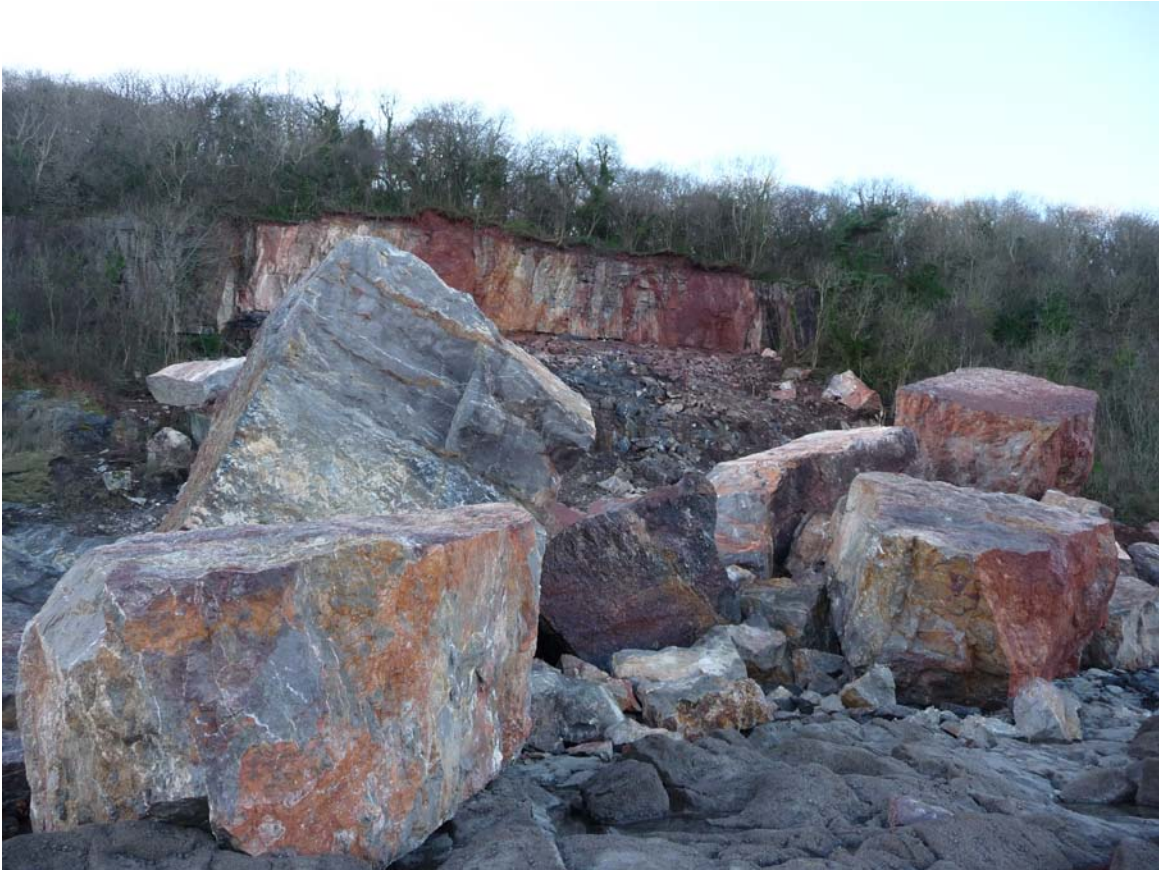
Figure 6. Close-up view of the Oxwich Bay landslide. Photograph taken from NGR 250710 185887 looking west.
