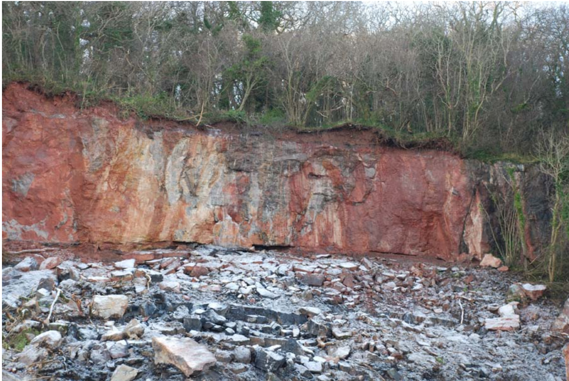
Figure 7. Close up of the back wall of the landslide. Red iron-oxide weathering caused by water percolation into former fracture. (Photograph courtesy of Mr P. M. Williams).
