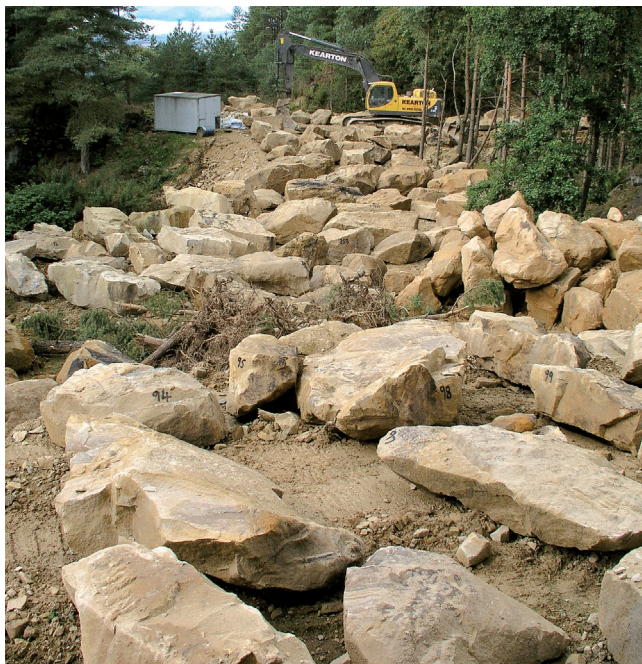
Blocks of sandstone stockpiled in Millknock Quarry awaiting processing
