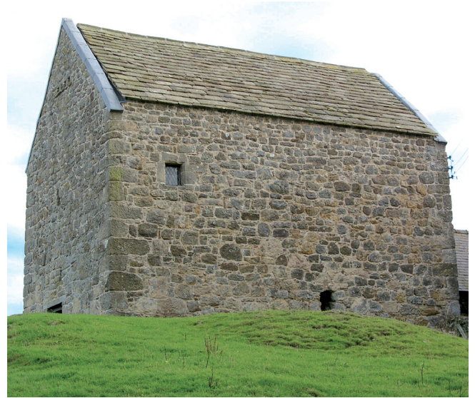
Hole Bastle, near Bellingham, constructed from random rubble sandstone with roughly dressed larger blocks used for corner stones and surrounds to openings. The flagstone roof is typical of those once common in southern parts of the district
