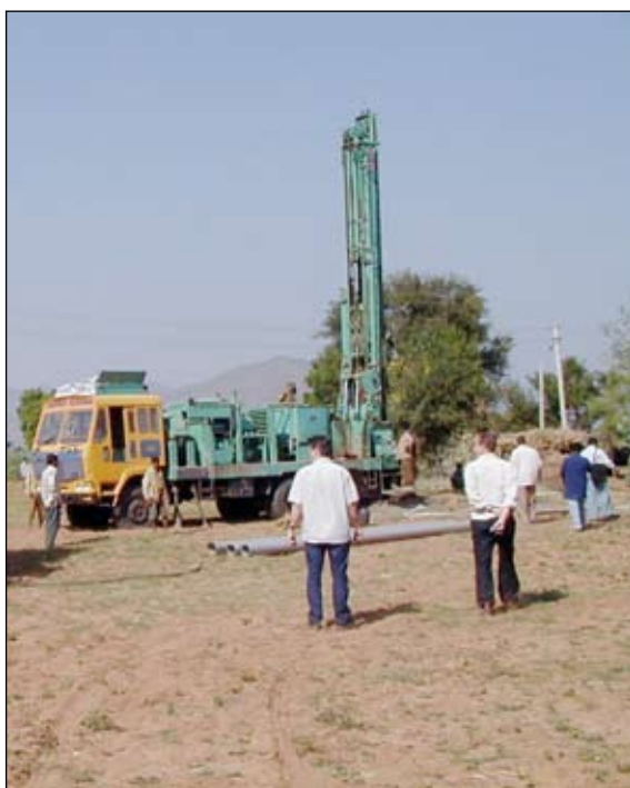
Photo A4.1 Drilling monitoring boreholes in the Satlasana research watershed.
