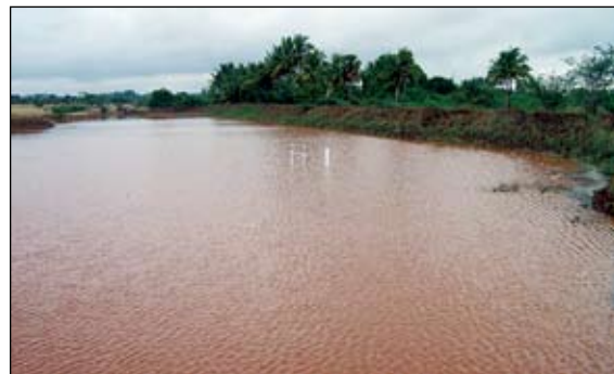
Photo A3.2 Automatic water level recording device in Karanampettai recharge structure when nearly full.
