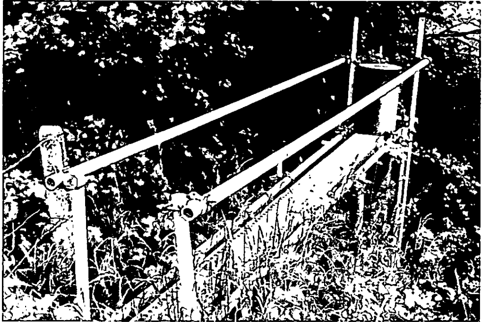
Plate 5.6 Stilling well - large gantry
