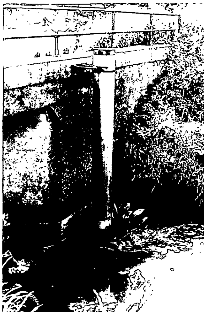
Plate 5.2 Stilling well - reinforced concrete bridge attachment
