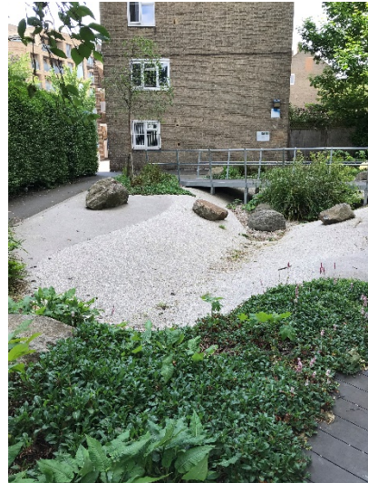
Figure 8. Low maintenance stony detention basin
