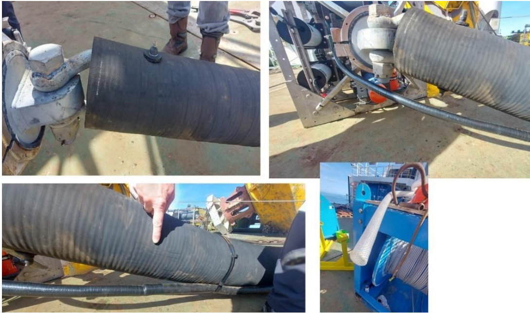
Pictures show how the chain cover was held in place by a bolt through the chain next to the frame shackle. The umbilical was attached to this and the coating lengthened using reinforced plastic tube that was covered with tape.
