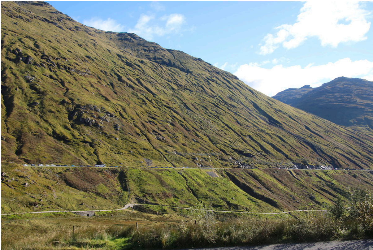
Fig. 2. Field picture showing the steep topography, the shallow landslides and the debris flows and their incisions above and the A83 at the Rest and Be Thankful pass. Note the cars and bus for scale. The upper road is the road for the public and the lower road is a military road. Source: David Petley on AGU blog ( blogs.agu.org/landslideblog/2020/10/09/rest-and-be-thankful/ ).
