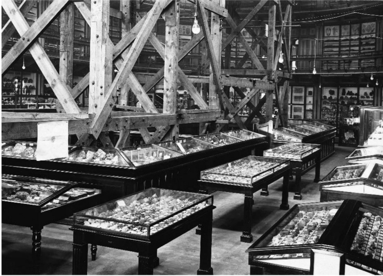
Fig. 12. Main floor of the museum with wooden scaffolding to support roof whilst cracked ironwork was inspected. Source: British Geological Survey, image no. P640471.
