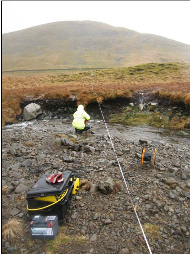
Figure 2: Installation of electrodes along ERT survey line at Talla Linnfoots facing north. Geophysicist in centre of image is installing an electrode in the stream bed
