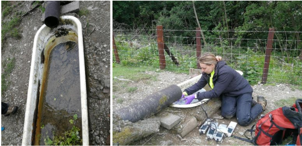
Figure 13 DG4, discharge and field parameters measured from outlet. The pipe is set into the hillside (uphill of a holiday park). No source could be traced further uphill, though a narrow patch of bulrush grows on the hillside for several metres above the pipe indicative of moist ground conditions.
