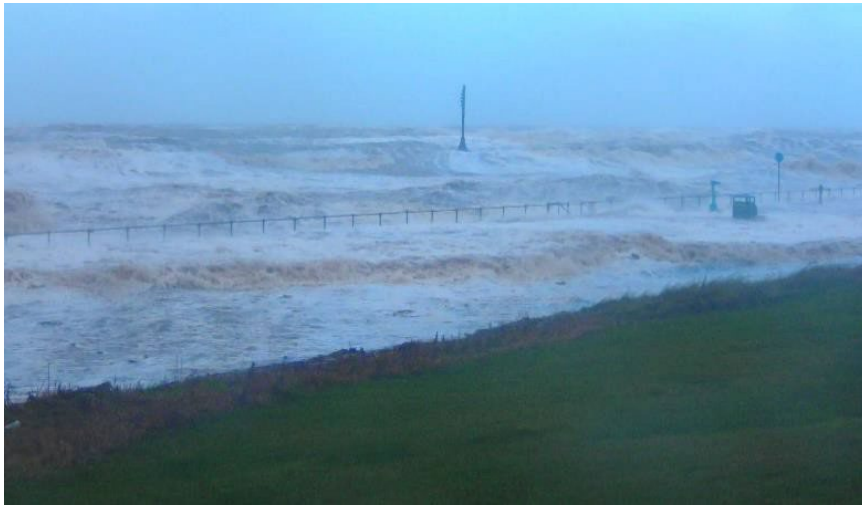
Figure 1. The Crosby sea wall frontage, 5 December 2013. Photo provided by the Sefton Council.
