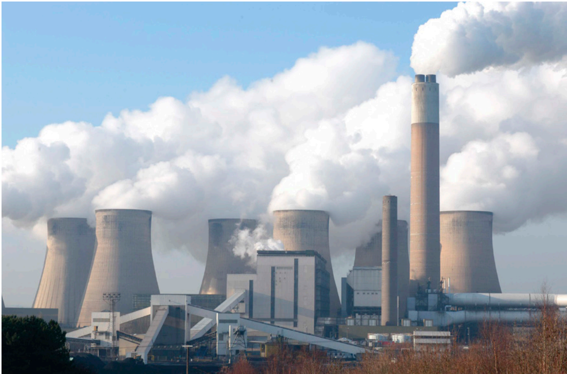
Ratcliffe-on-Soar coal fired power station and FGD plant (in foreground) ©NERC/BGS.
