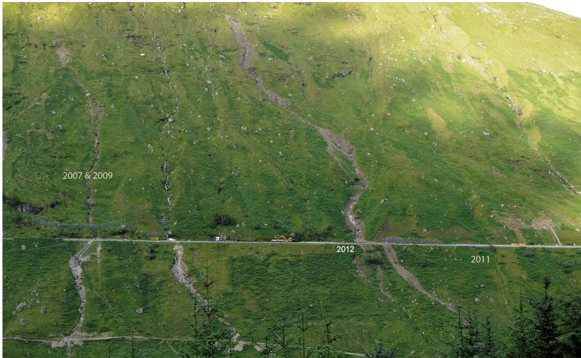
Figure 7 Recent debris flows on the A83 Rest and Be Thankful Pass BGS © UKRI 2012 P785411.
