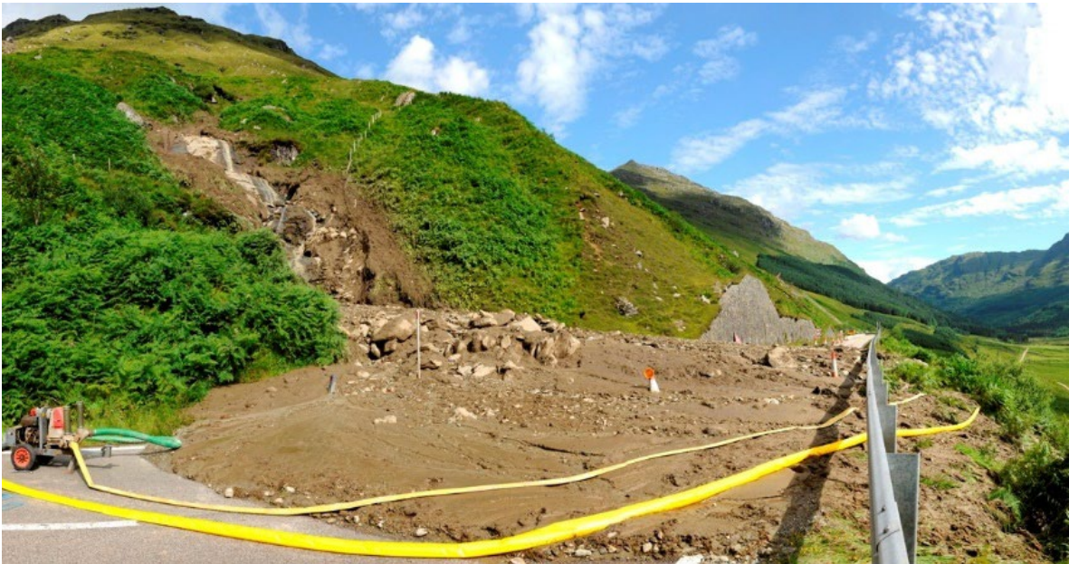
Figure 6 Debris flow deposit blocking the A83 Rest and Be Thankful, August 2012. BGS © UKRI 2012 P785430.
