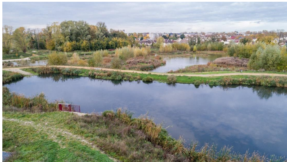
Figure 7. Newly created wetlands: river expands to a larger floodplain, thus preventing flooding in neighbouring settlement while providing habitats for many species © SIAH: Syndicat Intercommunal d’Aménagement Hydraulique of Croult and Petit Rosne.
