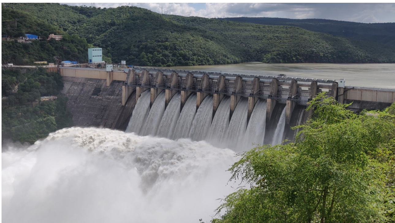
Srisailem Dam, Andhrapradesh (Photo credit: Garudachedu Vishnu, Shutterstock)
