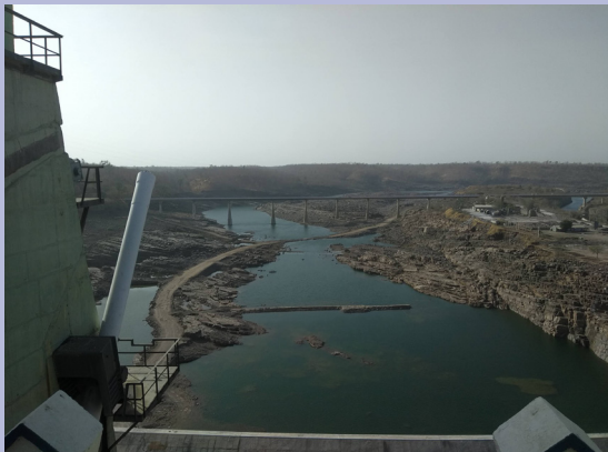
Indira Sagar Dam, Madhya Pradesh (Photo credit: Nathan Rickards)
