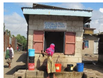
Water kiosk obtaining water from nearby borehole
