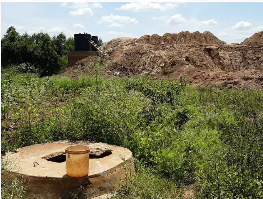
Figure 17 Private shallow well with tailings leaching plant using cyanidation visible in the background
