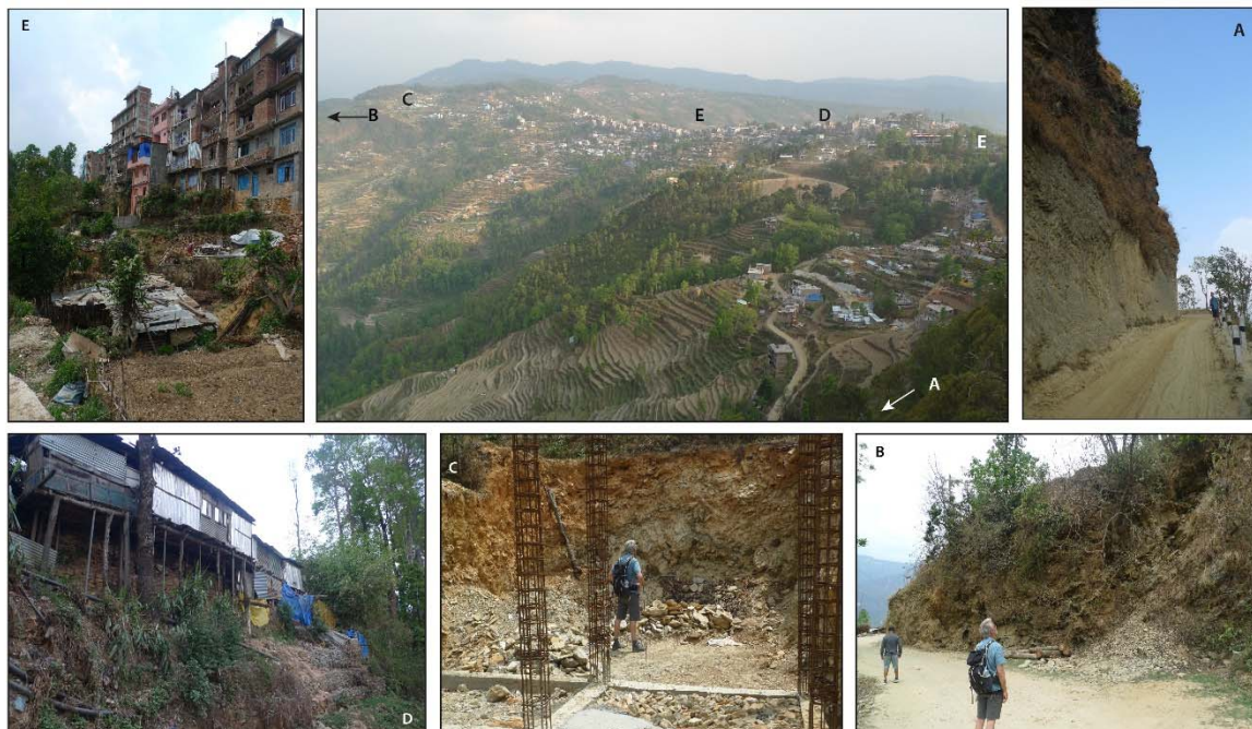
698 699 Figure 9. Central image provides a context for the ridge-top urbanised community of Chautara. (A) Vulnerable 700 and exposed access road beneath a steep rock wall to the north of the town. (B) An active landslide at the 701 southern edge of the town. Local people reported that the large block moves every monsoon and impacts the 702 road. (C) Conditions for excavating foundations are challenging. The surface material comprises weathered 703 and fractured bedrock, and has been affected by slope movement. (D) Informal housing at a slope edge, 704 illustrating the challenges of building where flat space is limited. (E) There is a lack of flat building space at the 705 town edge and buildings are constructed several storeys high at the slope edge.
