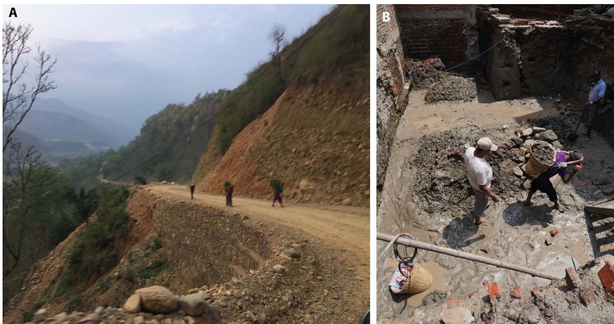
634 635 Figure 7. (A) The road that accesses communities on the Salyantar terrace is cut into a steep escarpment that is 636 vulnerable to instability during monsoon rains. (B) Excavation in silts and fine sands with a sump pump, for 637 building foundations in Bhaktapur in April 2018. Evidence for liquefaction below the feet of the construction 638 workers. Local people reported that this stage of reconstruction is not possible during the monsoon.
