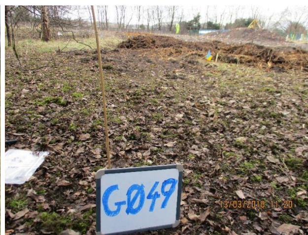
c) GGERFS03 with proximity of new car park works
