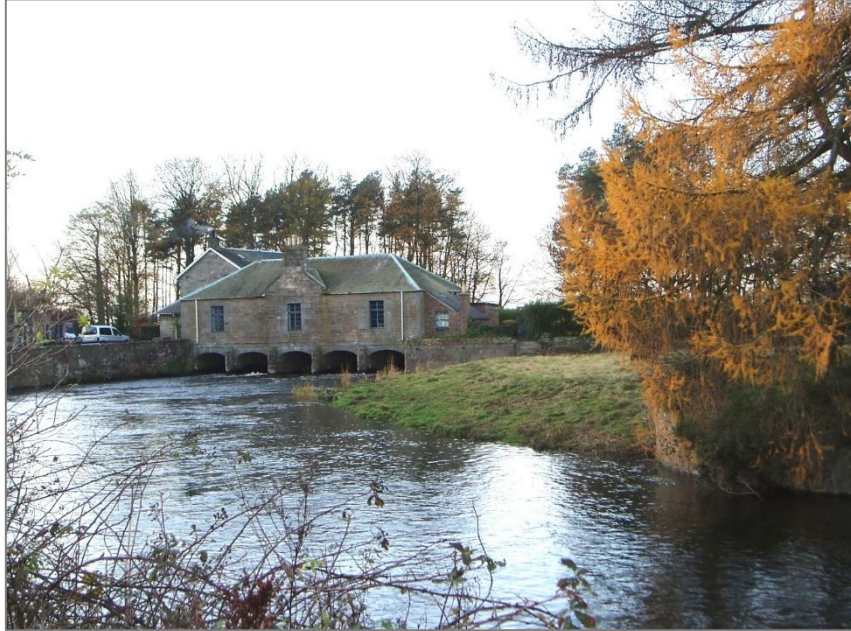
Figure 1 Sluice gates on the outflow from Loch Leven. (Photo: Linda May)
