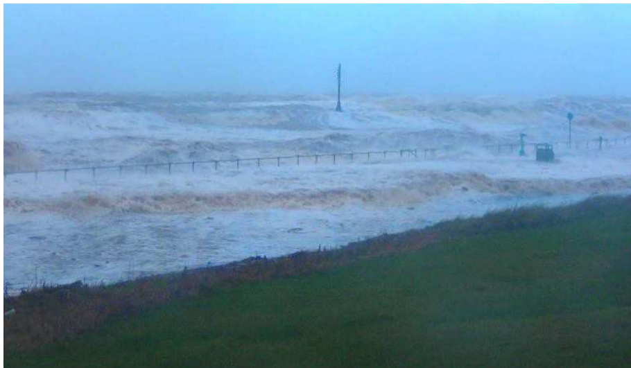
Fig. 1. The Crosby sea wall frontage, 5 December 2013. Photo provided by the Sefton Council.
