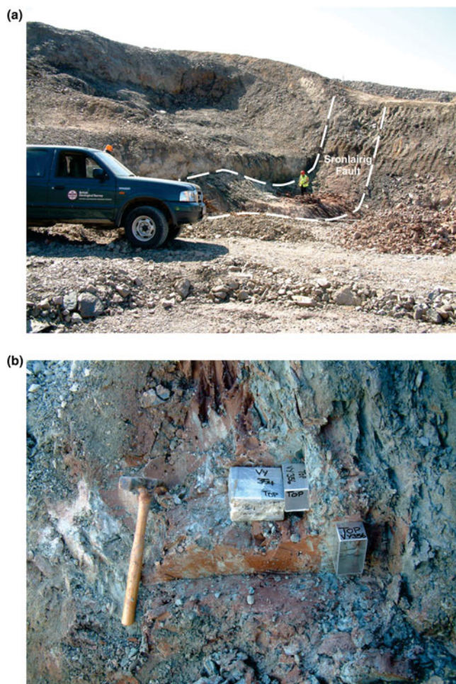
Fig. 2. (a) Sronlairig Fault exposed in the temporary excavations for the Glendoe hydroelectric dam plinth. View is looking to the southwest. (b) Kubiena tin sampling of the Sronlairig Fault gouge. The boundary between the dominantly grey–green and dominantly brown material is aligned ENE (centre-top) to the WSW (lower right-hand corner).
