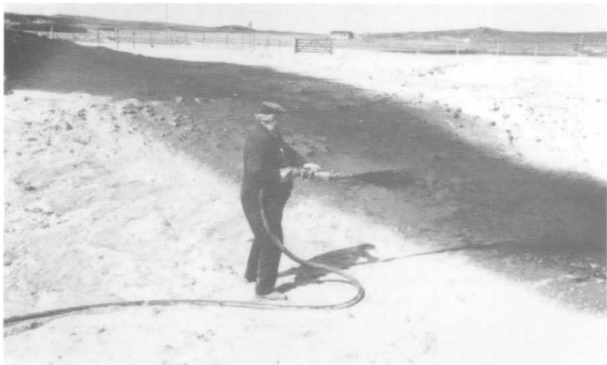
Plate 17. Hydraulic seeding at Mellon Udrigle, Ross-shire, Scotland. This method is useful in difficult sites where rapid stabilization is required, but it is expensive compared with traditional methods of sand stabilization. (Photograph W T Band, Countryside Commission for Scotland copyright)
