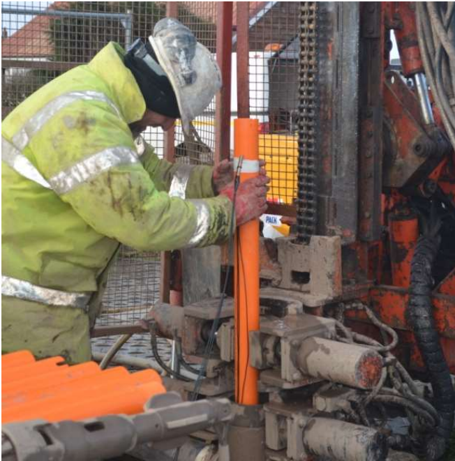
Figure 30 Inclinometer tube segment, with PRIME borehole resistivity array attached, being lowered in Borehole 3b
