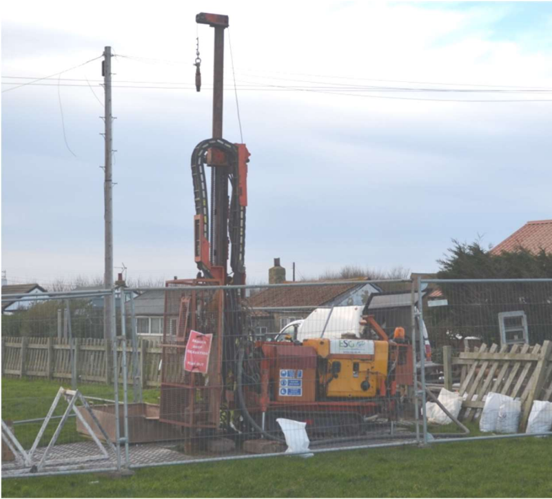
Figure 27 ESG's Beretta T41 drill on borehole 3b at Aldbrough
