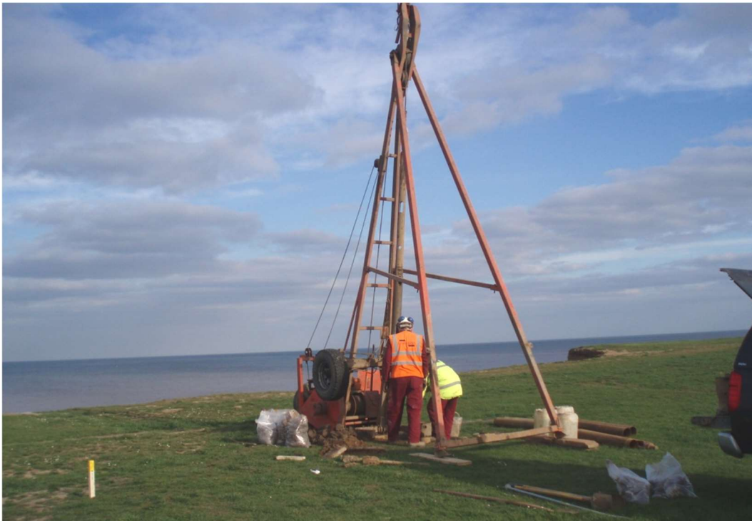
Figure 6 Cable percussion drilling rig at borehole 1a (Geotechnics Ltd.), 19 th March 2012
