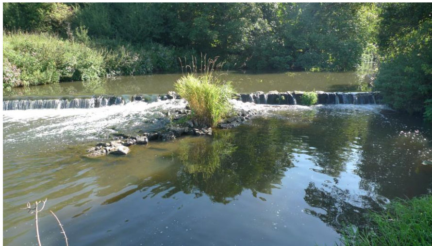
Figure 9. The lower weir (approximately 400 m downstream from Clerkington Weir), which was previously covered by alluvium, and has once more become exposed by channel migration.
