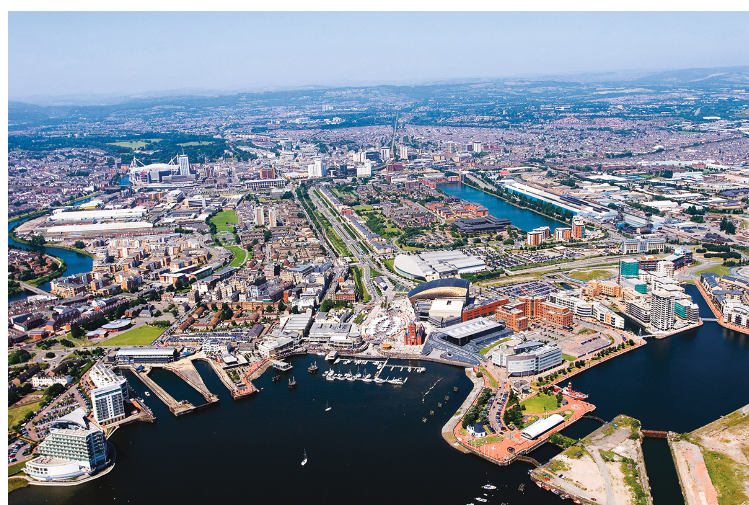
Fig. 1. Aerial view of coastal City of Cardiff which has an urban population of 300,000 and plans to build 40,000 new low-carbon homes. (Photo courtesy of Cardiff City Council)
