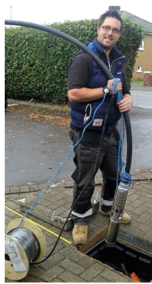
Fig. 5. Installation of borehole water pump.
