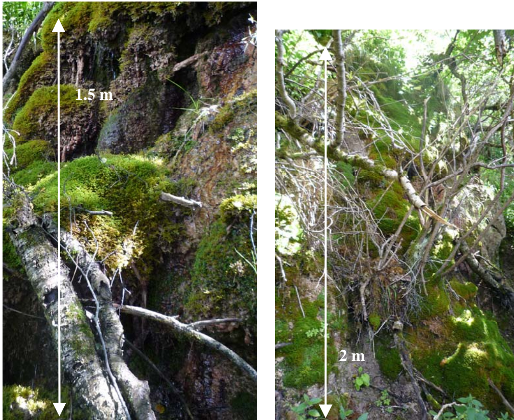
Figure 8 Multiple small spring flows (seeps) over areas of rock face, covered with vegetation
