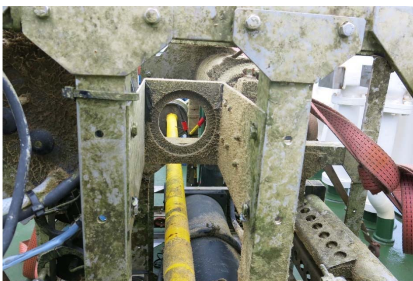
Figure 20 - The slot where the Seaguard (S/N 1130) was initially located. The growth on the inner ring of the bottom clamp suggests it had been lost for some time
