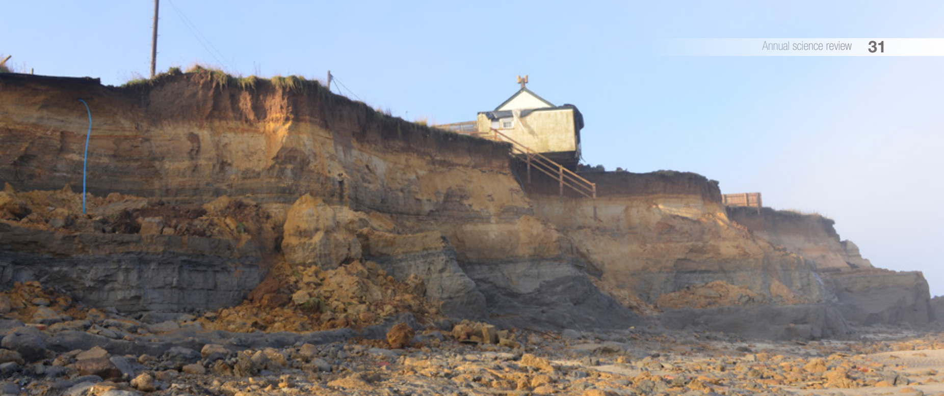
Cliff erosion at Happisburgh, Norfolk, after the December 2013 storm surge.
