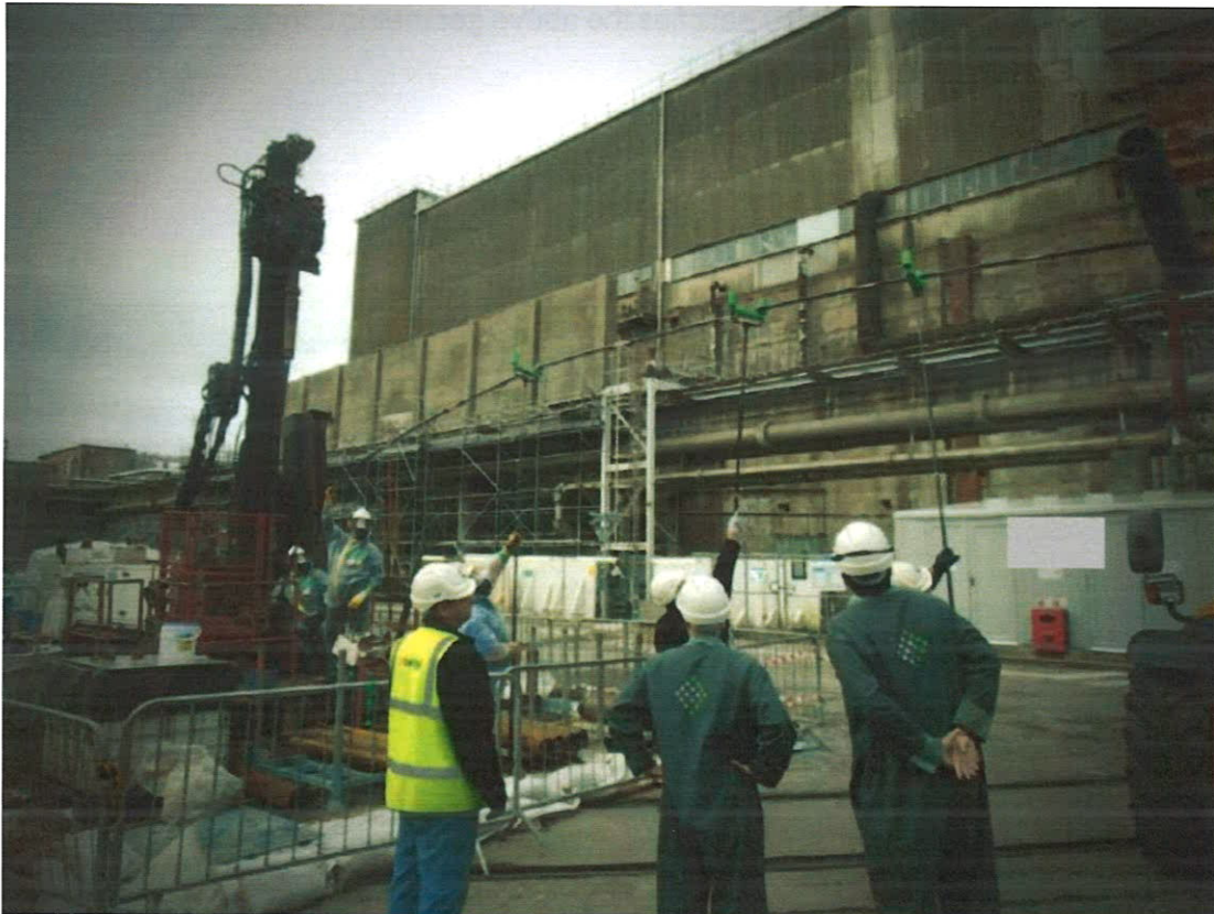
Fig. 2. ERT borehole installation at MSSS.
