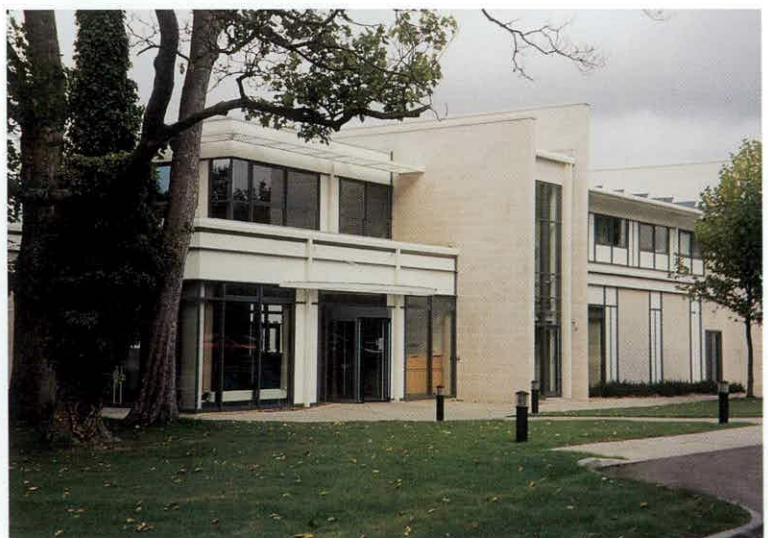
The new extension to IH at Wallingford completed in Spring 1999 as part of NERC's Rationalisation & Restructuring Programme.
